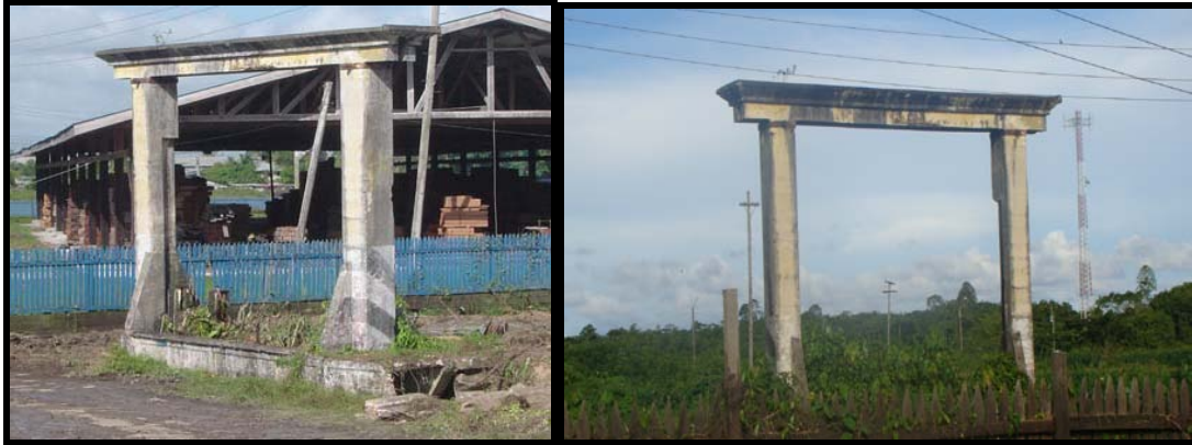
Figure 2.4 River Sluice to be reactivated
