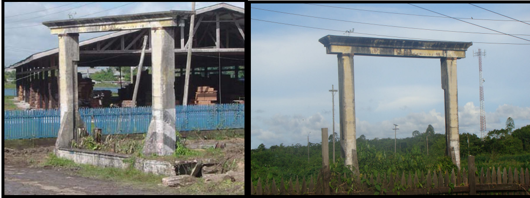
Figure 2.4 River Sluice to be reactivated
